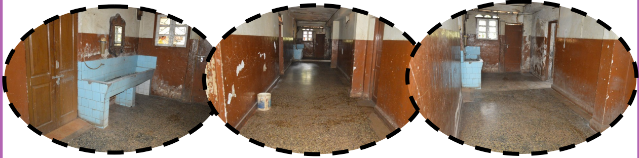
Stage 1: Before the work began
