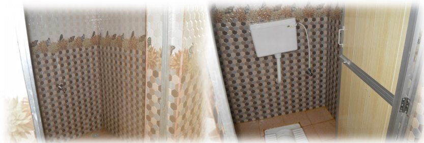
Stage 3: After the work is done!
