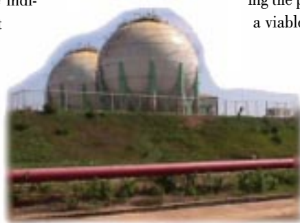
PNOC: an eco-industrial park in the making
