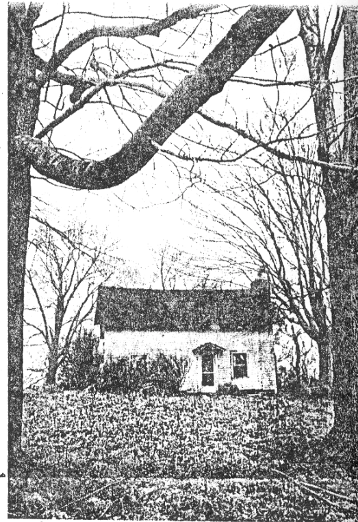
BENEATH THE OLD WEATHERBOARDING on this house at Spice Knob is the 20 by 40 foot log house built by Felty Husk, Daviess County's second settler, sometime around or prior to 1810. The National Endowment for the Arts has granted the Owensboro Area Museum $8,050 (to be matched by the Junior League of Owensboro) to move the house to the Kentucky Wesleyan College campus and restore it to original shape. (Staff photo by Bill Welch)
