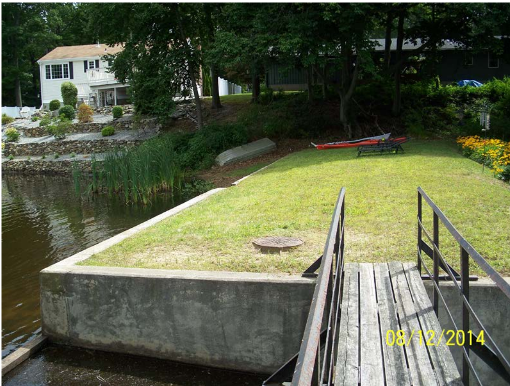
Photo 5a – An overview of the dam crest from the right abutment looking towards the left. The spillway footbridge crossing is in the foreground, and a manhole cover just to the left of the bridge and past the spillway training wall is the outlet valve control chamber.
