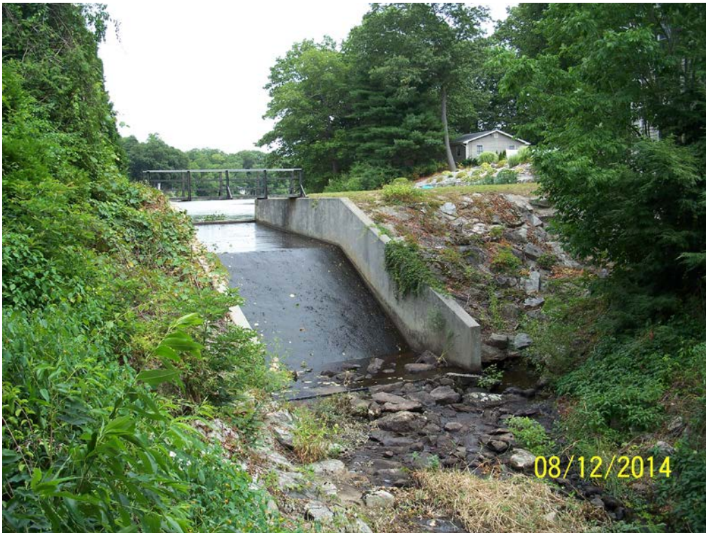
Photo 21f – Another view of the dense vegetative cover along the right and left embankment and toe areas.
