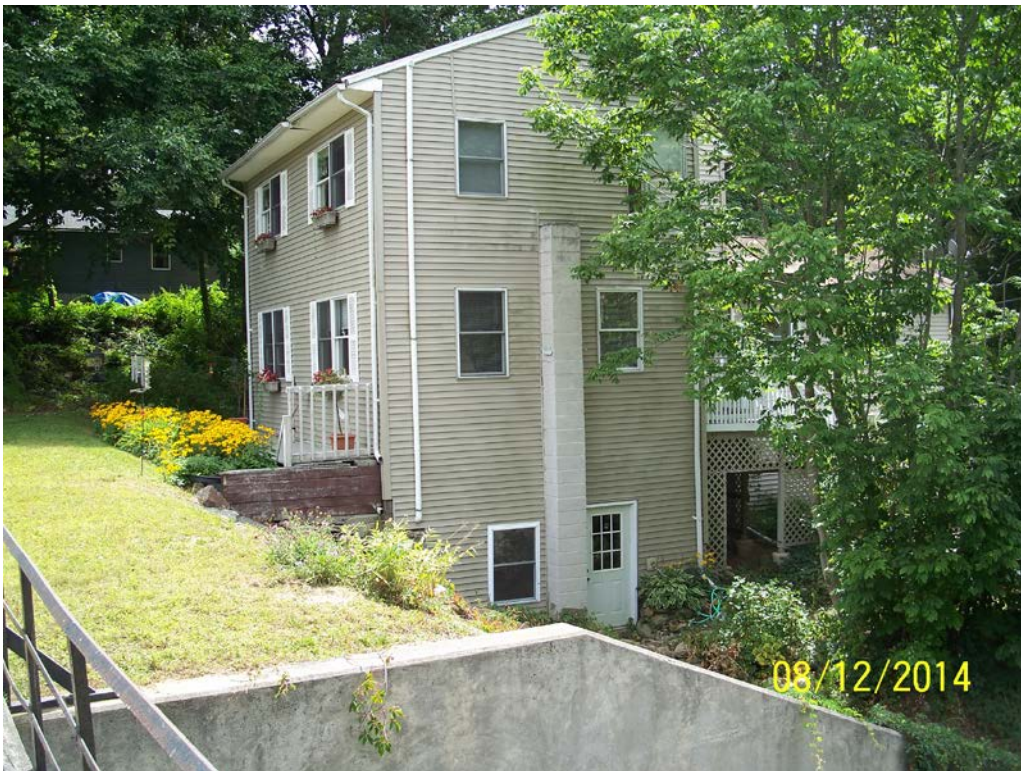
Photo 7b – The downstream face left of the spillway, showing growth of small trees along the left toe area.
