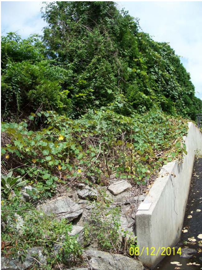
Photo 11a – Overview of the right training wall with dense brush and arbor vitae growth.
