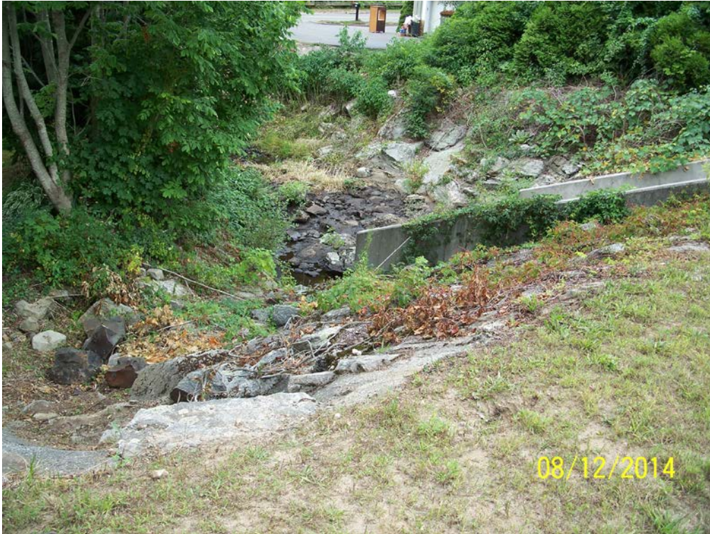
Photo 21e – An overview of the left downstream embankment, toe and channel areas, showing tree, brush and woody vegetative growth.
