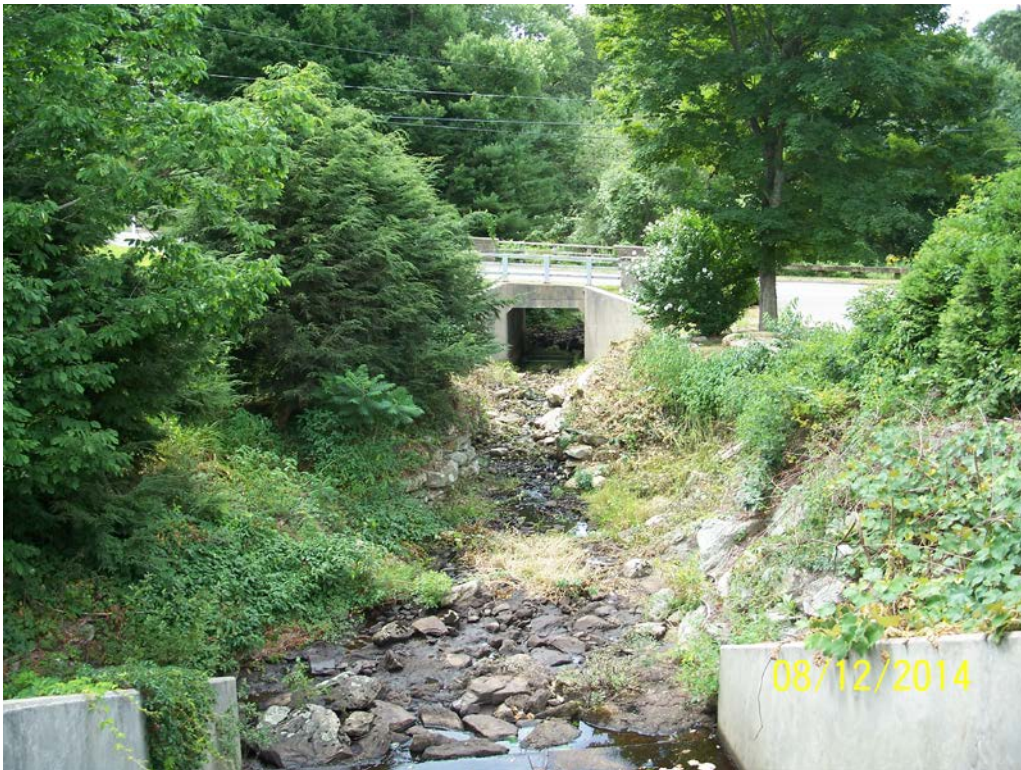
Photo 15b – An overview of the downstream channel as seen from the top of the spillway looking toward the road culvert. Note dense vegetative growth along the channel slopes.
