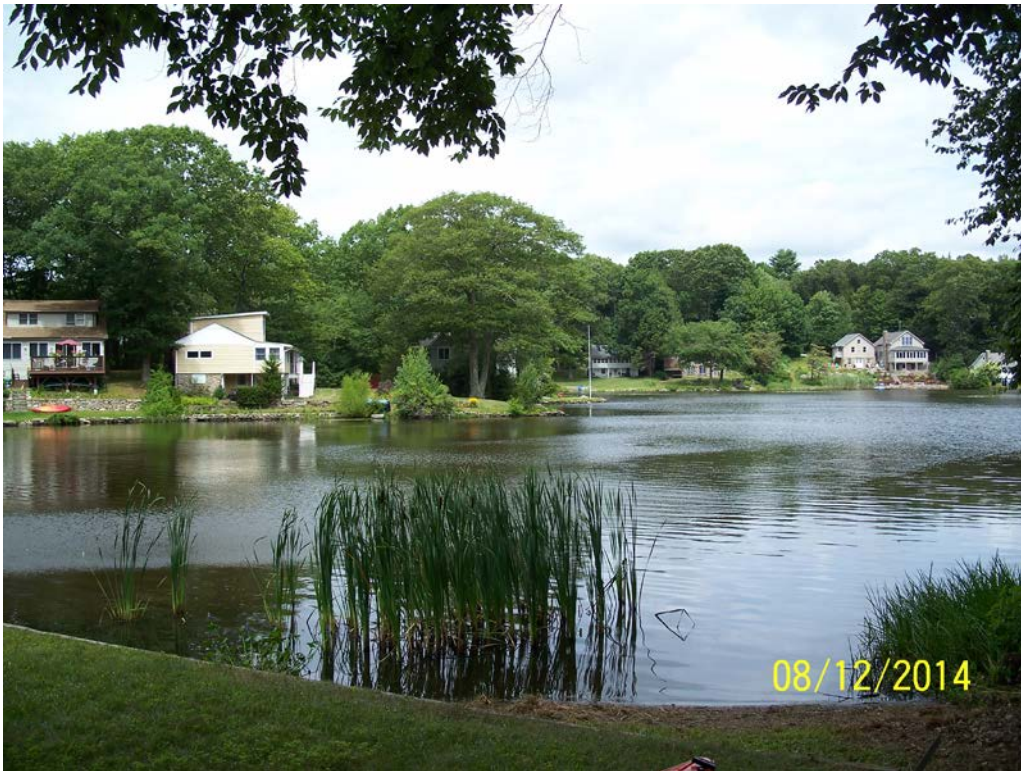
Photo 20 – An overview of Hidden Lake as seen from the left abutment of the dam.
