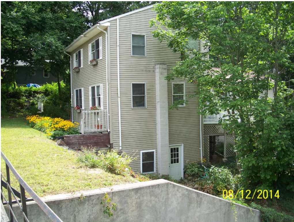
Photo 5b – Another overview of the dam from the right abutment showing the relationship of the downstream house to the dam embankment.
