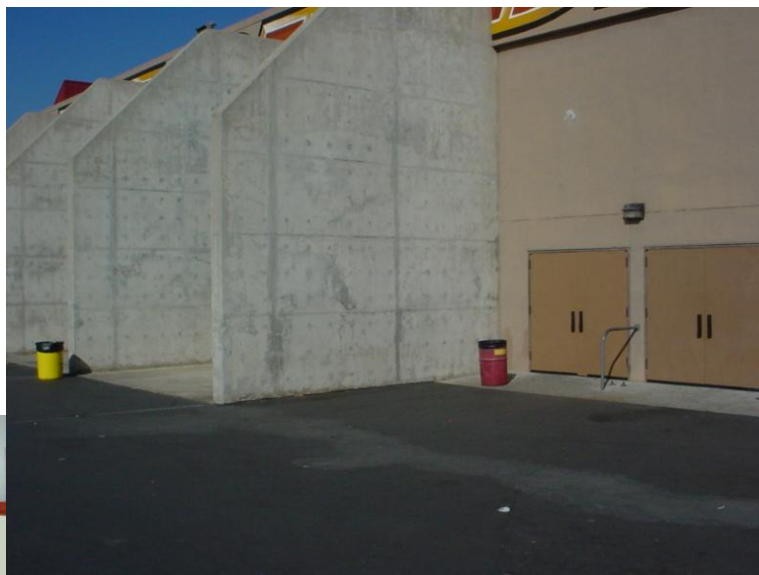
Staging area outside the gym.
