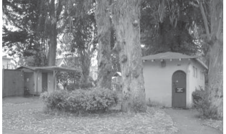
Maintenance will always be the main challenge for Panhandle toilets.
